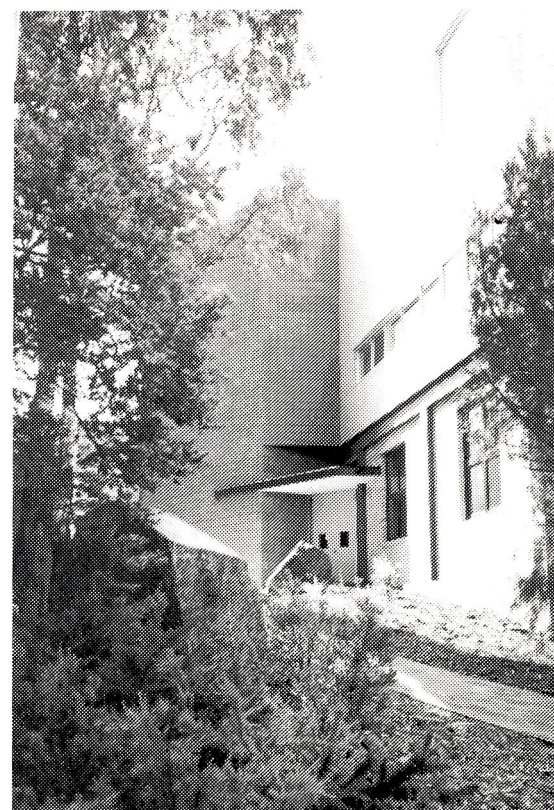
The recently completed second-floor extensions to the CODES building.
